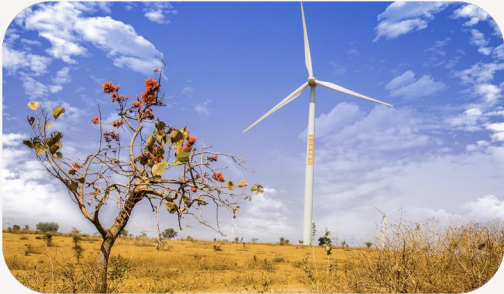
Using wind power in Madhya Pradesh, India
