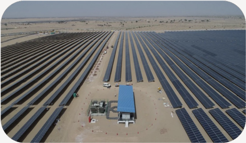
Using solar energy in Bhadla, Rajasthan, India
